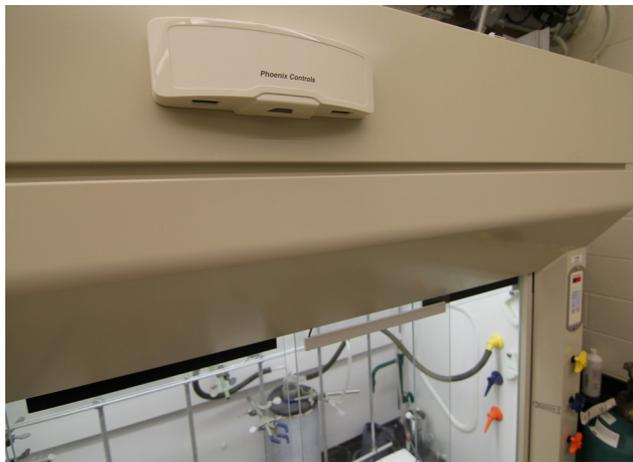
Fume hoods were decommissioned and new Phoenix Controls ZPS sensors and fume hood monitors (FHM) were installed, allowing the hoods to scale back to unoccupied ventilation levels automatically.
