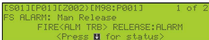
Figure 10-6 Interlock Release In Alarm After Two Minutes Sitting Idle
