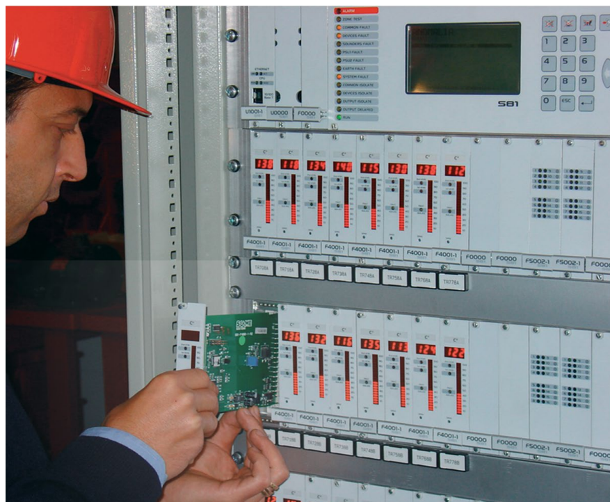
Hot swap of cards and power supplies with no need for panel shutoff
