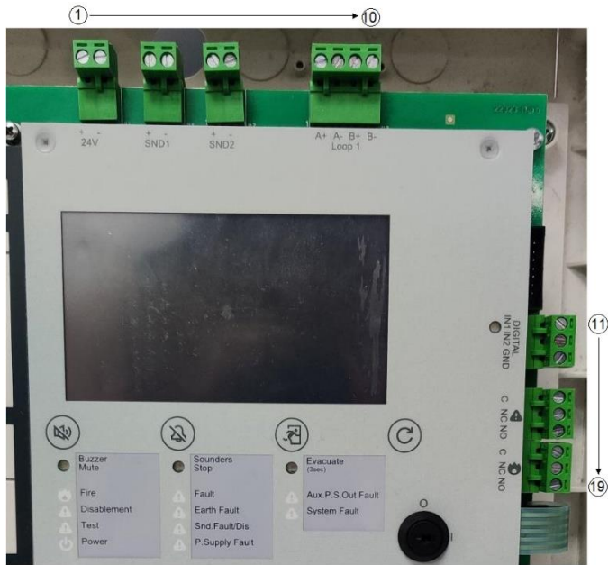
Fig. 16: Main Board connector sequence
