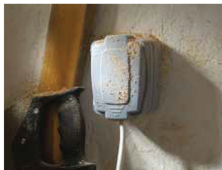
Dust proof connection to safeguard work areas.
